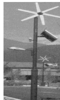
Fig 6: PV Light System Combined With Small Wind Turbine [11].
