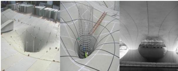
Fig. 1: EPS Formwork [5, 6]
