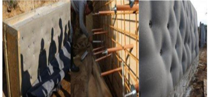
Fig. 3: Textile Formwork [12, 13]
