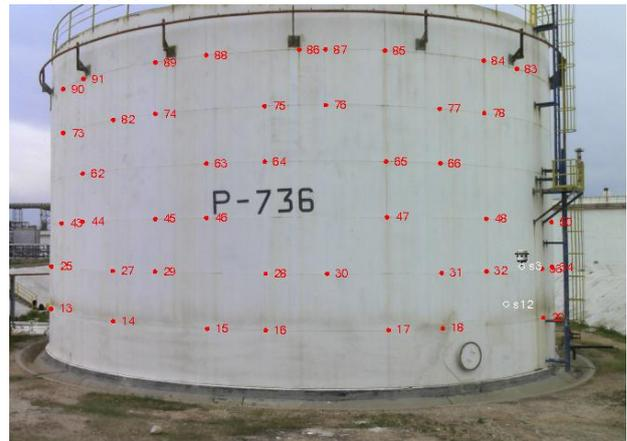
Fig 9. The six horizontal cross sections on the tank's shell.
