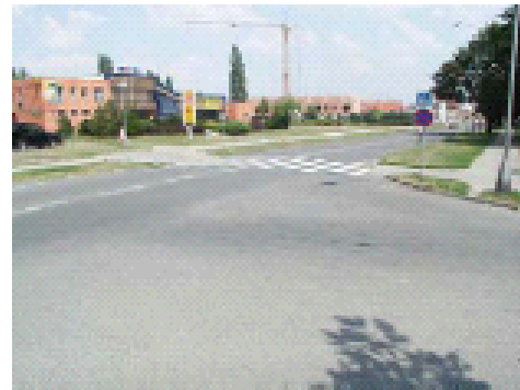
Fig 6-3: Crossing is too long
