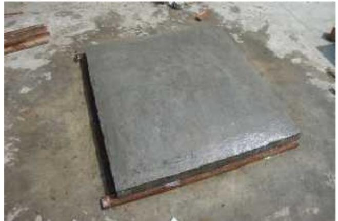
**Fig.10. Removing of edge beam mould**
