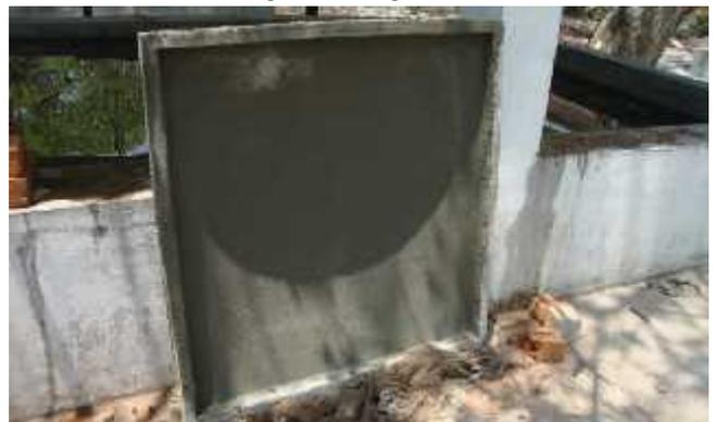
**Fig.11. Finished funicular shell**
