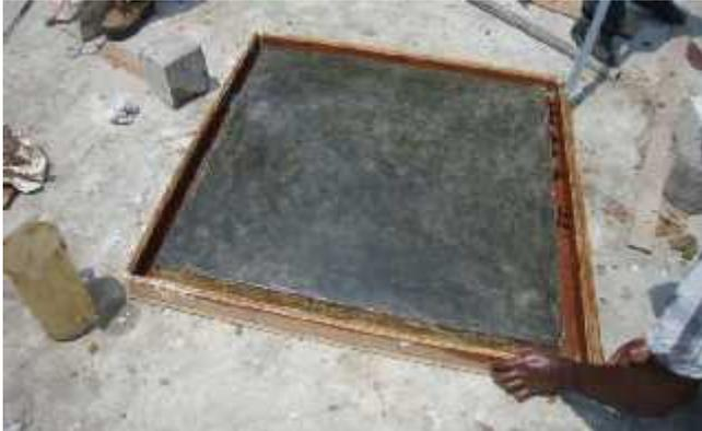
**Fig.6. Fixing outer mould for the shell**
