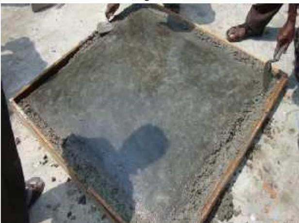
**Fig.8. Casting of edge beam**
