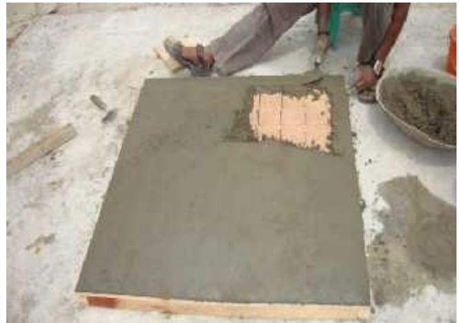
**Fig.4. Finishing the surface with cement mortar**
