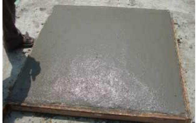
**Fig.9. Finished shell Surface**
