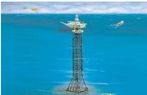
(Fig.-2 Amerada Hess Compliant Tower at Baldpate Garden Banks (First freestanding, non-guyed compliant tower installed in 1998)
