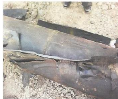
Fig 5.Casing Removal under progress
