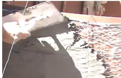
Fig. 2 – Ferro cement technic to build water reservatory in northeast of the Brazil
