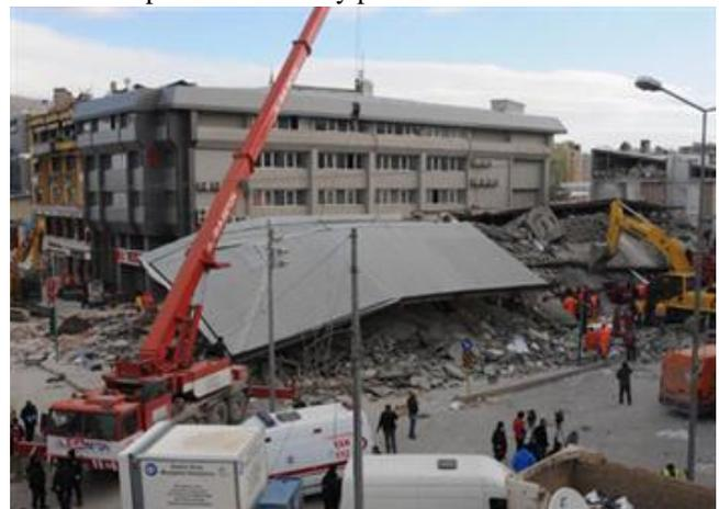
**Fig. 1** Collapse down to its foundations of the Bayram hotel during the second earthquake of Mw=5.7 in the city of Van (Turkey) on 9 November 2011 (courtesy of E. Lekkas).
