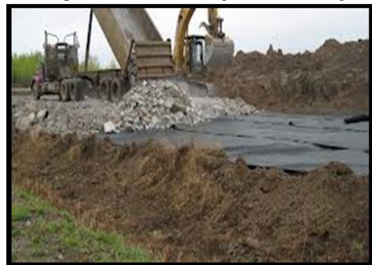
Fig. 4 Pre-Fabricated Asphalt Membrane Lining
