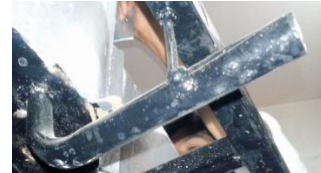
Picture 4: Water Drain
