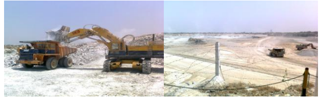
Loading the raw material
