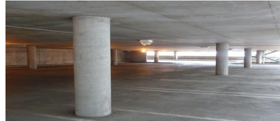
Fig 1: Typical flat slab construction
